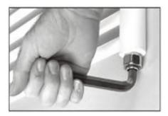
3. Attach valve and by hand and turn it to the correct position then tighten using an appropriate tool, usually a spanner.
